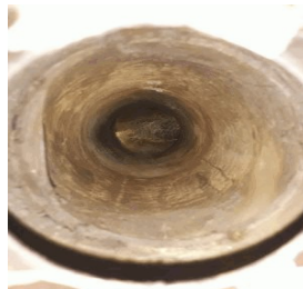
toilet ducting after
