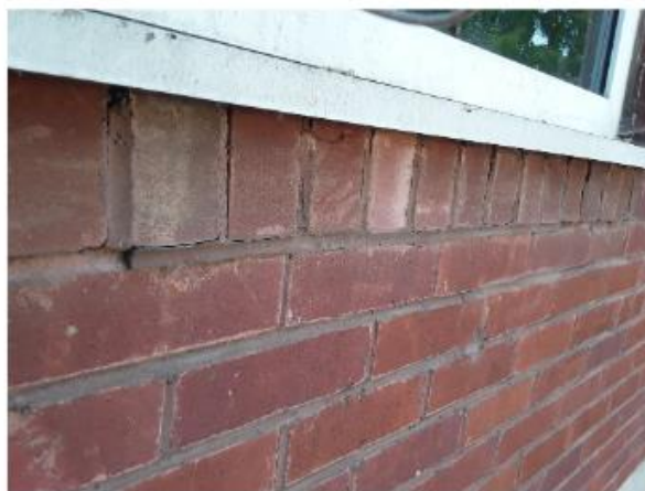
Photo 134 – Defect EEE19, Bulging brickwork, mortar surface degraded, and area of vertical cracks in mortar, 3 no. cracks, <2mm wide
