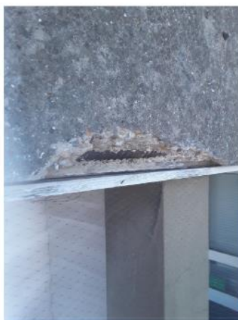
Photo 503 – Defect EWE01, Spalled concrete, material removed during survey
