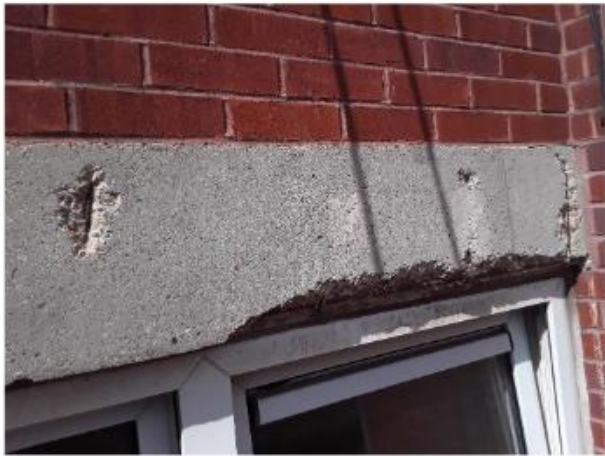
Photo 99 – Defect EED02, Area of concrete spalls, 4 no. spalls, <100mm wide, area of previous repair, material removed during survey
