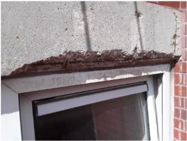
Photo 100 – Defect EED02, Area of concrete spalls, 4 no. spalls, <100mm wide, area of previous repair, material removed during survey
