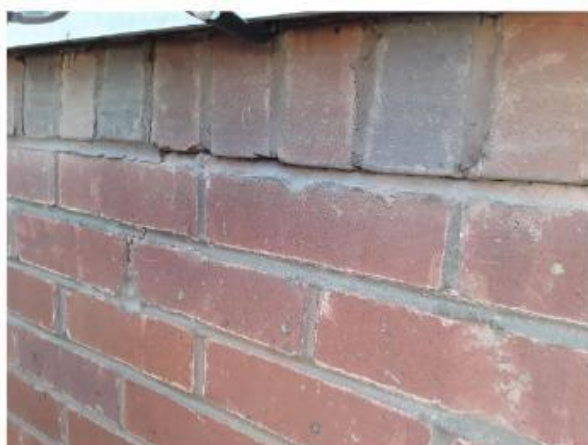
Photo 133 – Defect EEE19, Bulging brickwork, mortar surface degraded, and area of vertical cracks in mortar, 3 no. cracks, <2mm wide
