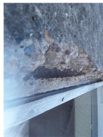
Photo 504 – Defect EWE01, Spalled concrete, material removed during survey
