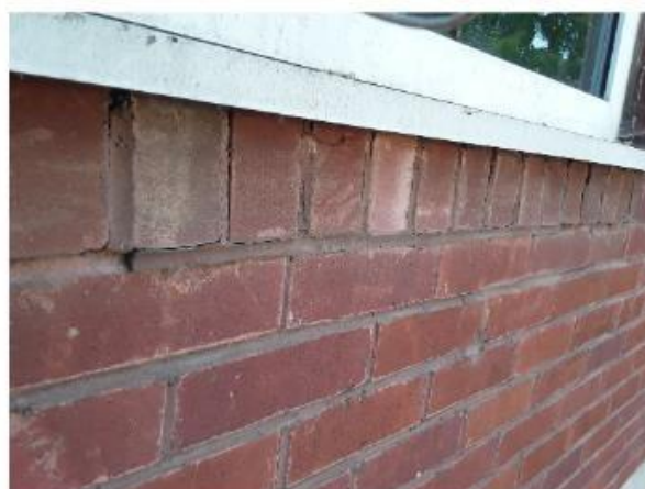
Photo 134 – Defect EEE19, Bulging brickwork, mortar surface degraded, and area of vertical cracks in mortar, 3 no. cracks, <2mm wide
