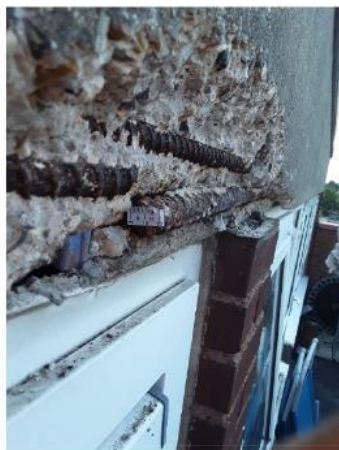
Photo 671 – Defect EWU01, Spalled concrete, material removed during survey
