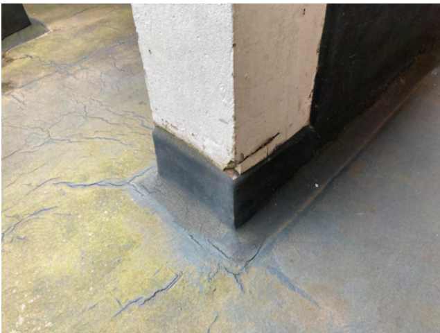
Photo 3.15: Crack in base of column on 4 th floor walkway in front of sub entry to flats 252-257
