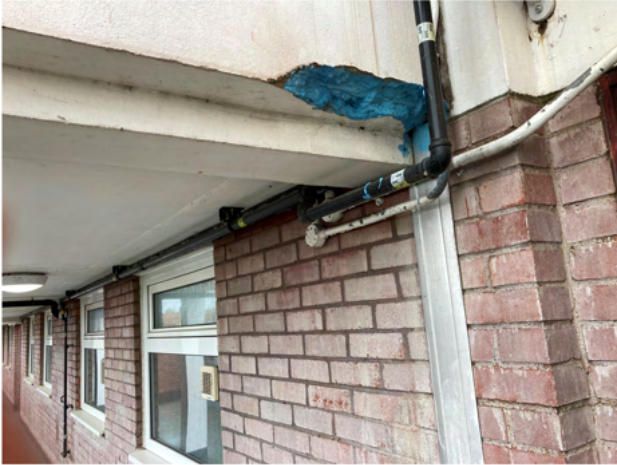
Photo 3.21: Severely spalled concrete with surface painted. Adjacent to entry to flats 177-182 at 4 th floor walkway. Same beam in photo 22.
