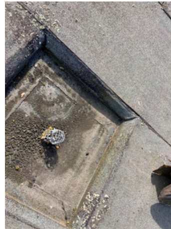
Photo 3.2: Filth around drainage inlet
