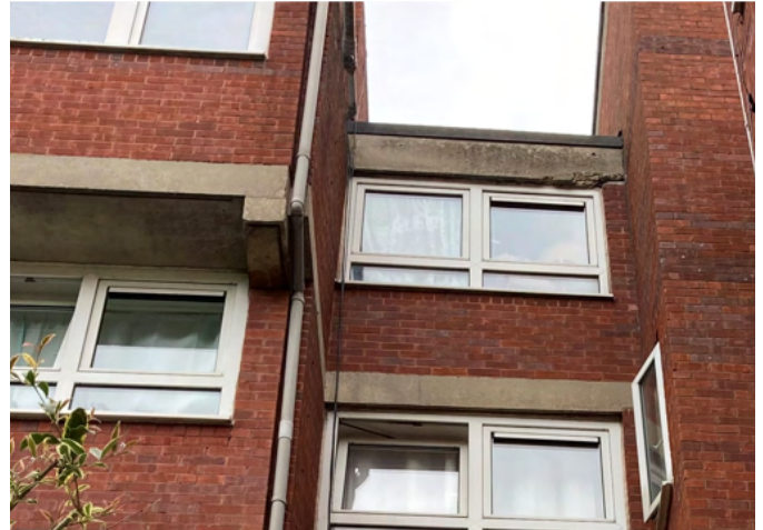
Photo 3.26: Spalled concrete in bottom corner of top lintol in recessed bay facing inner green above flat 127
