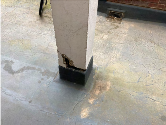
Photo 3.17: Crack and spalling of concrete at base of column in front of sub entry to flats 249-251 on 4 th floor walkway.
