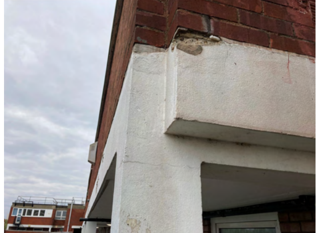
Photo 3.22: Spalling of concrete at top corner of beam. Same beam in photo 21
