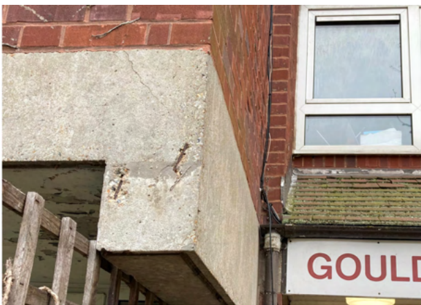
Photo 3.37: Spalling of concrete and diagonal top crack in beam LHS of Entrance B on Bullen Street
