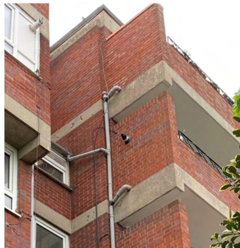
Photo 3.28: Cracks in recessed bay on 4 th and 5 th floor slab/beam faces adjacent downpipe between Flat 77 and Entrance B on Bullen Street
