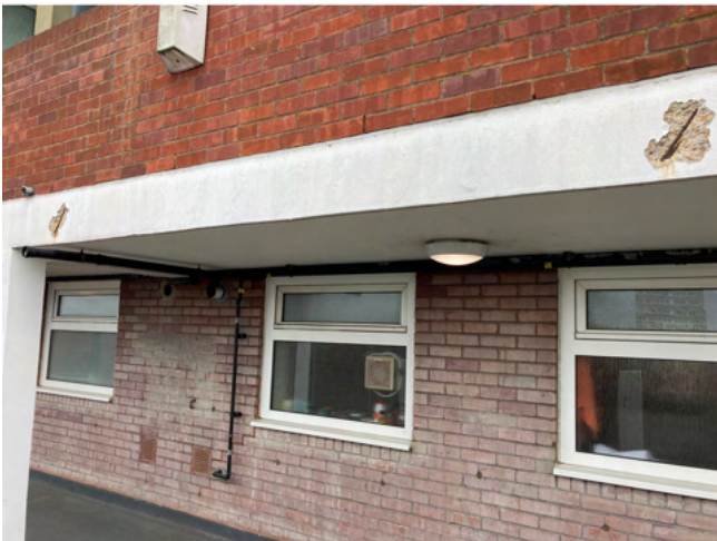
Photo 3.23: Spalling on 5 th floor slab edge visible from 4 th floor walkway between entry to 177-182 and 183-188
