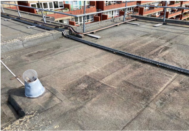
Photo 3.1: Roof surface showing evidence of rainwater ponding
