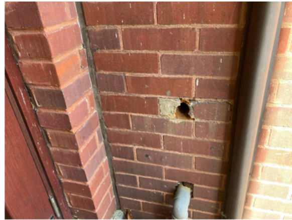
Photo 3.30: Entrance side wall to flat 44 facing inner green showing hole in brickwork resulting from pipe removal.
