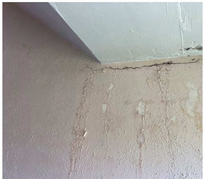
Photo 3.8: Sloped Roof over stairs to sub entry to flats 247-248: Horizontal crack in wall beneath slab. Evidence of moisture ingress.
