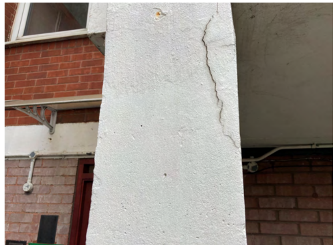
Photo 3.16: Crack at the top of column in front of sub entry to flats 249-251 on 4 th floor walkway
