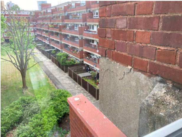
Photo 3.13: Crack in top corner of beam facing green adjacent stairwell to flats 208-209. Visible from landing window.
