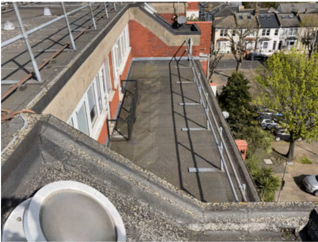
Photo 3.3: 5 th floor Communal Balcony Evidence of rainwater ponding
