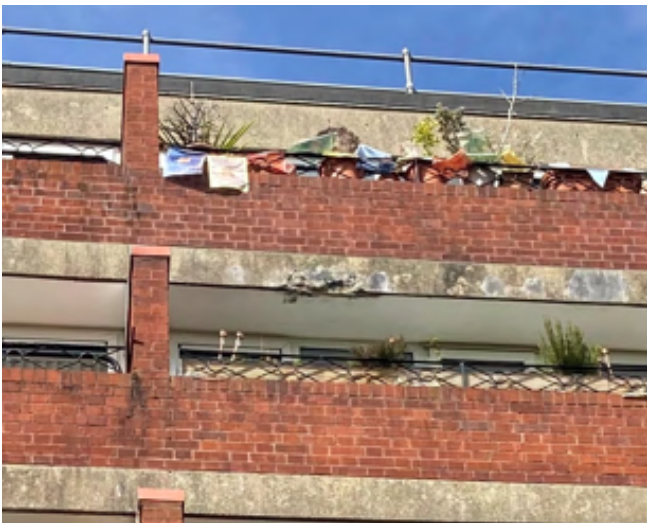
Photo 3.11: Spalling of concrete at bottom of 5 th floor balcony slab and roof beam facing inner green between sub entry to flats 37-38 and 44-43
