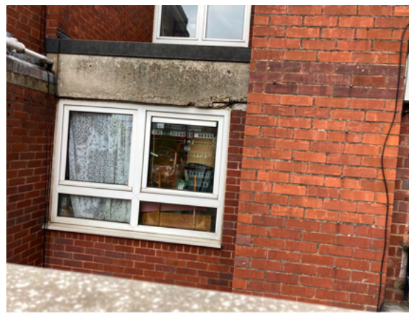
Photo 3.38: Concrete spalling at bottom RHS corner of lintol over storage window
