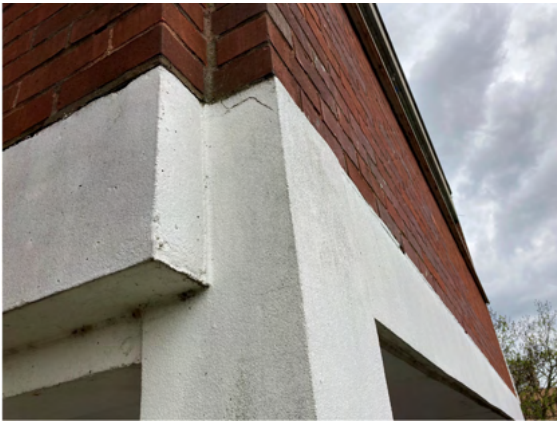
Photo 3.39: Crack at top corner of column on 4 th floor walkway adjacent to entrance to flats 264-269
