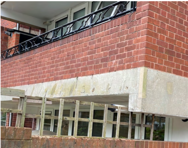
Photo 3.27: Multiple cracks on face of concrete slab at 1 st floor, LHS of Entrance C on Bullen Street
