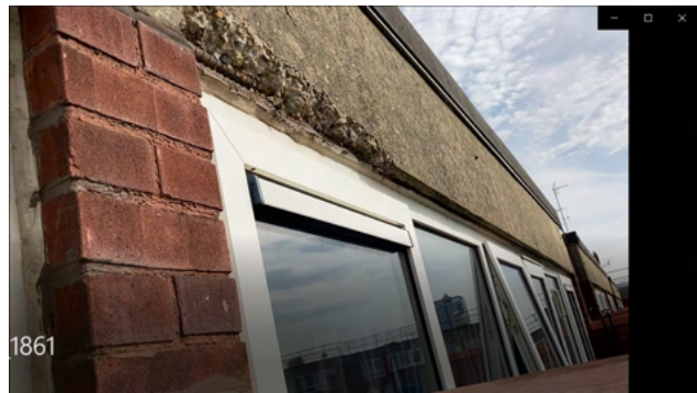
Photo 3.32: spalled concrete underside of balcony lintel in flat 187.
