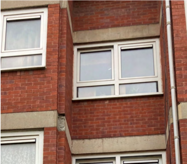
Photo 3.9: 2 nd floor slab adjacent flats 128 and 129 Loss of concrete at slab recess leaving brickwork unsupported.
