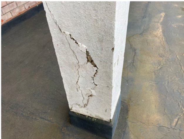
Photo 3.19: Column fractured at bottom on 4 th floor walkway, adjacent entry to flats 165-170
