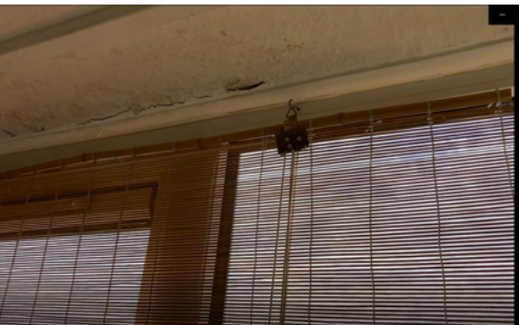
Photo 3.31: Peeling of paint underside of roof slab in living room of flat 182
