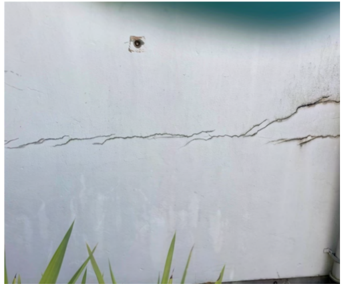
Photo 3.6: 4 th Floor Communal Terrace opposite flat 232 showing crack in side wall
