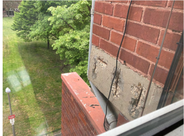
Photo 3.14: Spalling of concrete on beam surface exposing reinforcement, facing green adjacent stairwell to flats 216 and 217. Visible from landing window.
