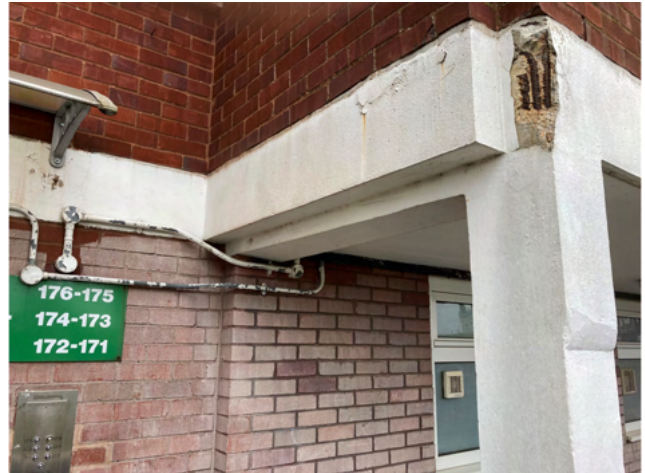
Photo 3.20: Severely spalled concrete exposing reinforcement at beam and column joint on 4 th floor walkway adjacent entry to flats 171-176
