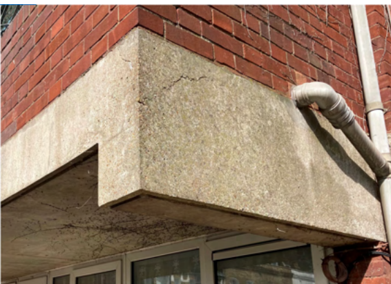
Photo 3.33: crack in repair work to concrete beam in the past
