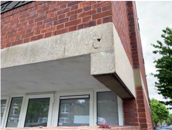
Photo 3.29: Cracked and spalled concrete on face of 1 st floor slab at corner of Bullen Street and Shuttleworth Road junction.
