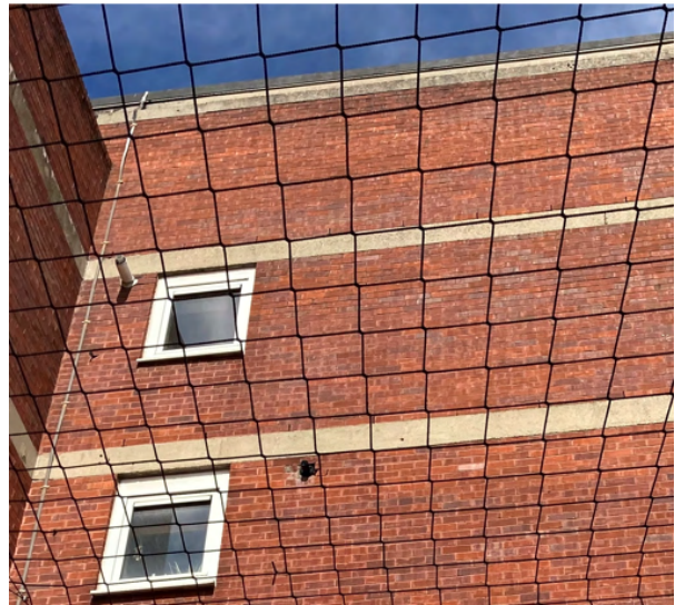
Photo 3.10: Side elevation facing Ball Court showing hole in brickwork underside of 4 th floor slab.
