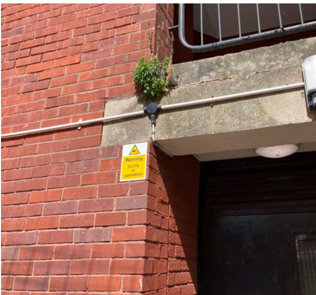
Photo 3.7: 5 th floor side elevation adjacent Ball Park. Vegetation growth
