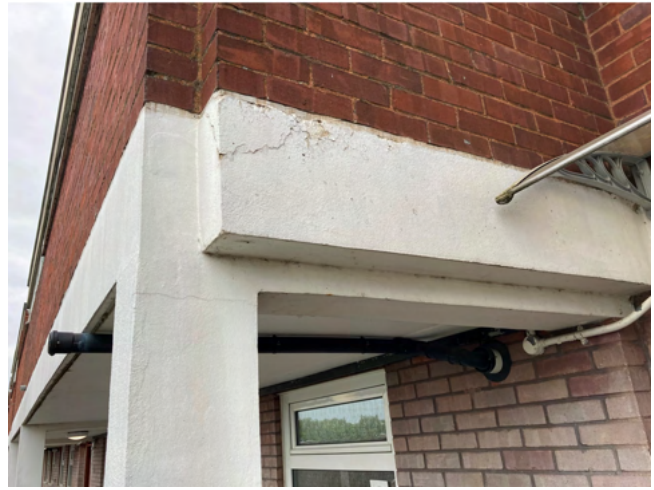
Photo 3.18: crack at top corner of beam LHS of entry to flats 165-170 at on 4 th floor walkway.
